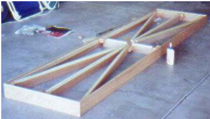
Figure 12: One 2x8-foot section of the platform, with all eight T-beams in place, is ready for the 1/4-inch plywood surface to be laid on top.
